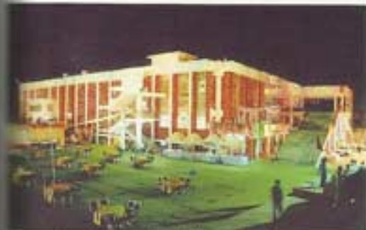
A captivating view of the auditorium
